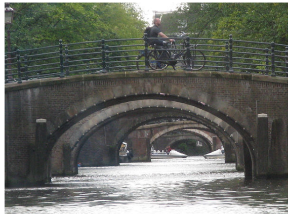
Bridges over a canal.
