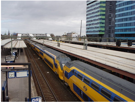
Arnhem Railway Station, Netherlands
