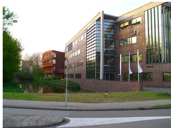
Site at business park “Delftechpark”
