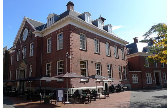
The (now monumental) former building of the Boerenleenbank in the Raiffeissenstraat (in the Centrum).
