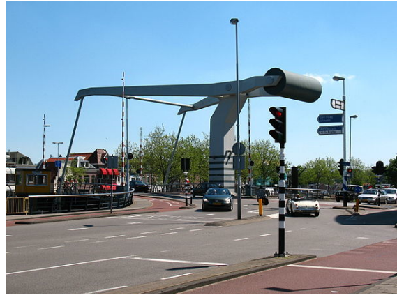
Lange Brug (Long Bridge), in popular speech also known as “de verfroller” (“the paint roller”).
