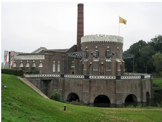
Pumping Station Cruquius
