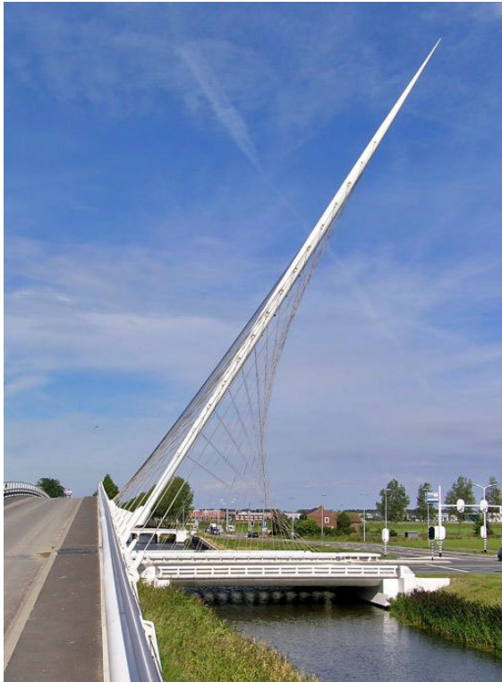
Calatrava bridge - Cittern
