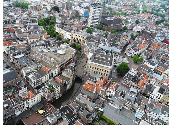
Aerial view of Utrecht from the Dom Tower
