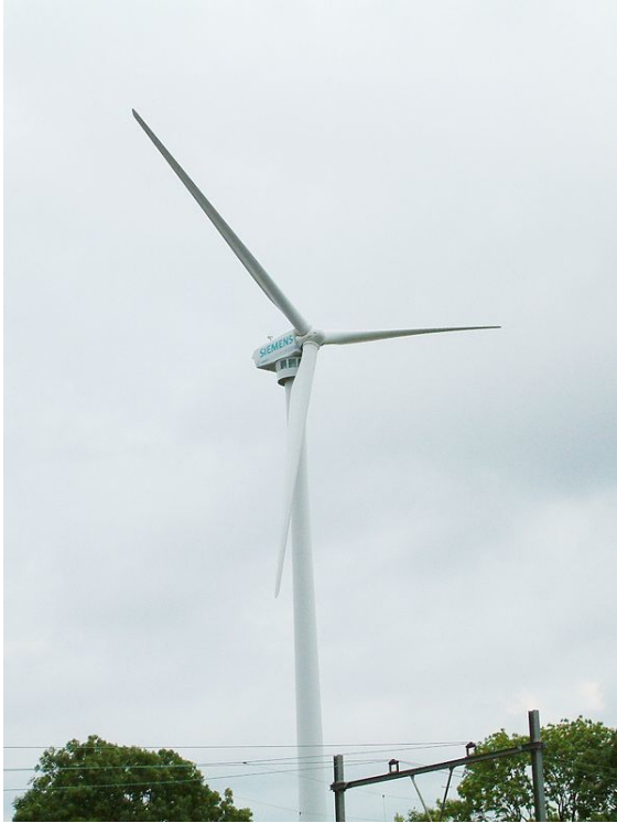
Wind turbine with observation deck at Siemens factory in Zoetermeer
